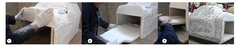
Step 8. Make sure to add insulation in the bottom of the oven.
