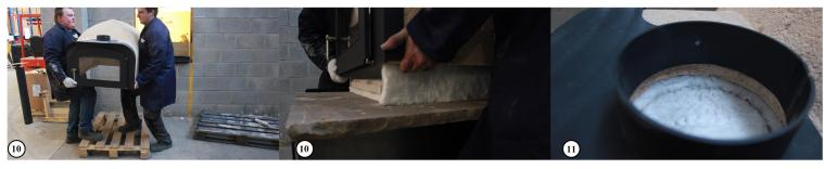
Step 11. Using the flue, score the insulation that covers the escape.Step 12. Then use a sharp knife to remove the covering insulation.Step 13. Place the flue back in and screw in place.
